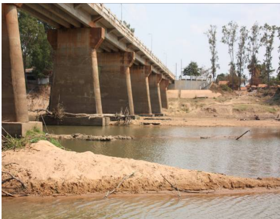
Sandan Bridge, 168m, across over Stung Sen River.
